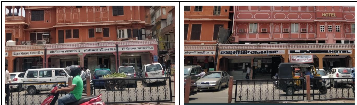
Inappropriate signages that have been combined
